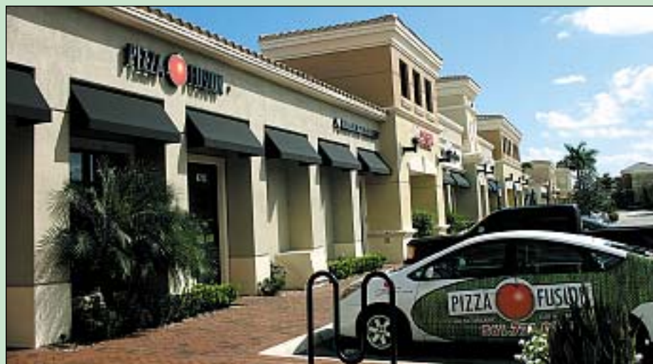
The Residences at Midtown is a mixed-use community featuring shops, a 500-seat cultural center, 300-seat banquet hall and several restaurants.
